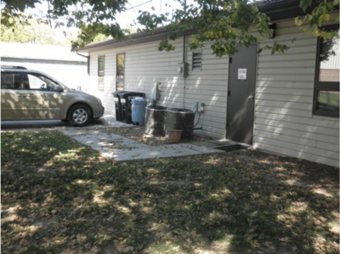
South Julie Street entrance designated for employee and emergency use only.
